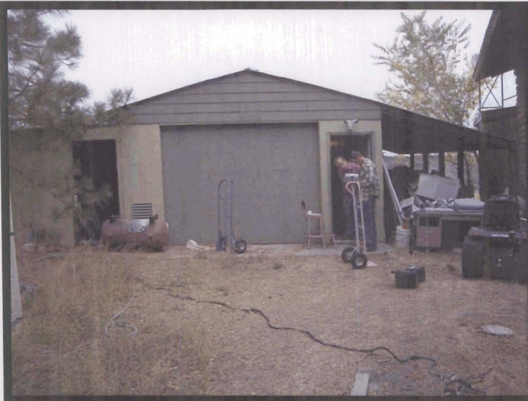
Shop #1 uses well to heat.
