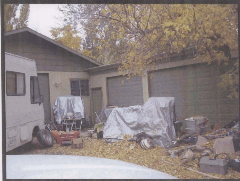
Shops #2 and #3 also make use of the well for heating.
