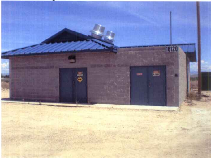
Well 13 Pump House
