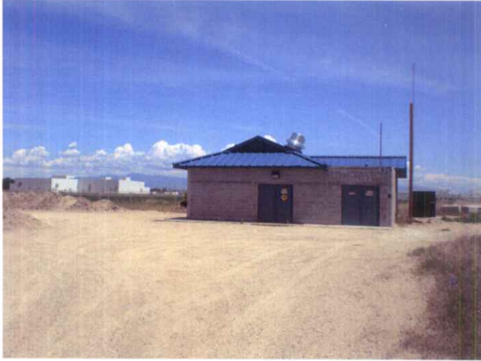
Well 13 Pump House
