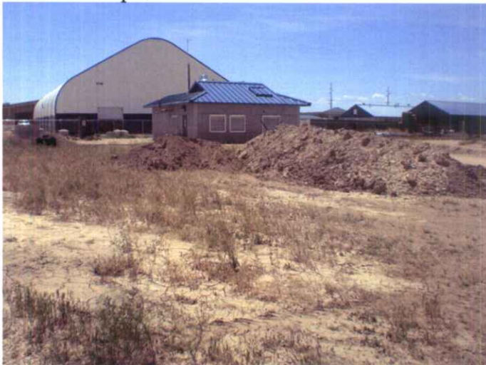
Well 13 Pump House
