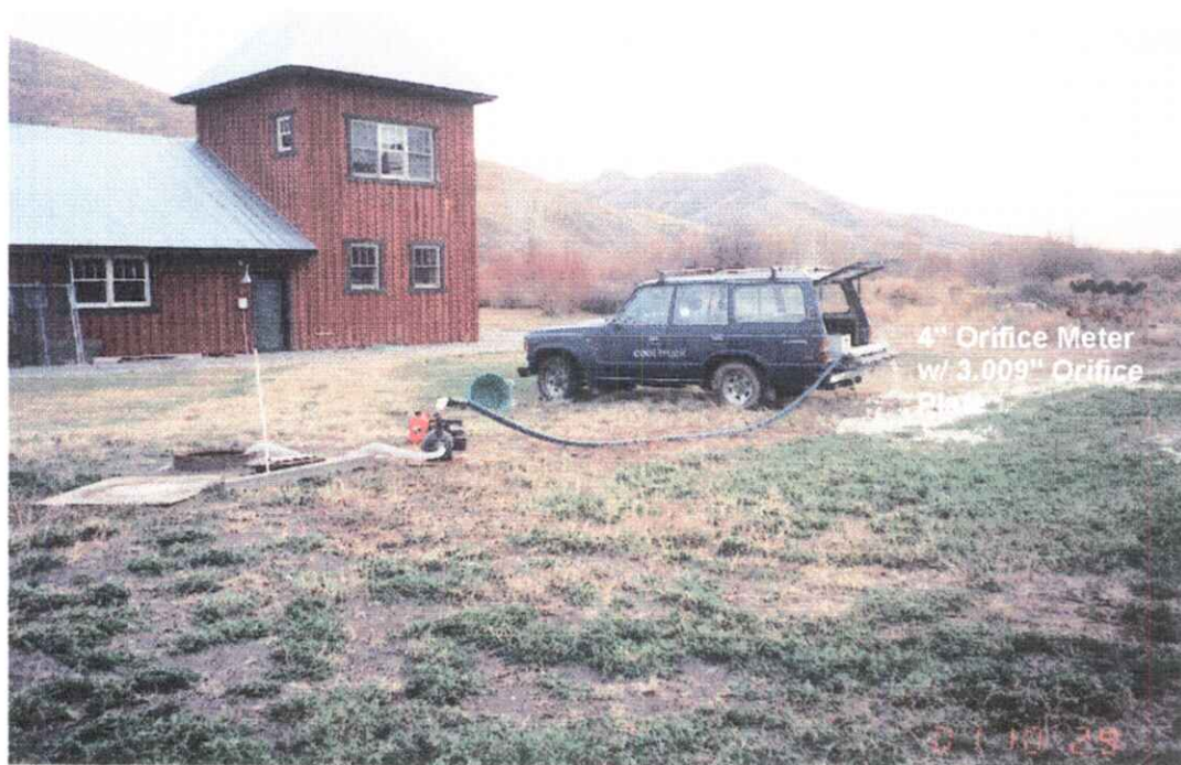
Pumping sump to determine system capacity.
