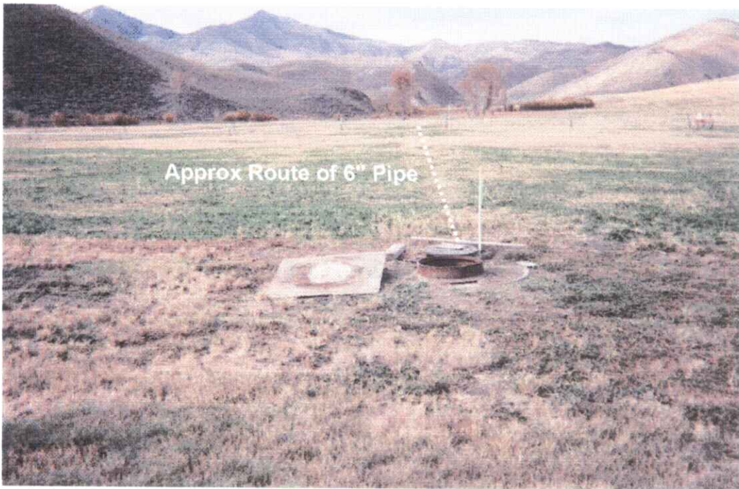
Hot Water Sump at End of 6" Delivery Pipe
