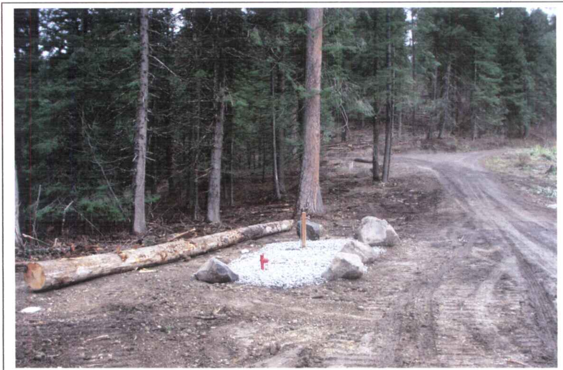
Photo 3: 11-17-2004 Spigot & Hydrant. Project completed.
