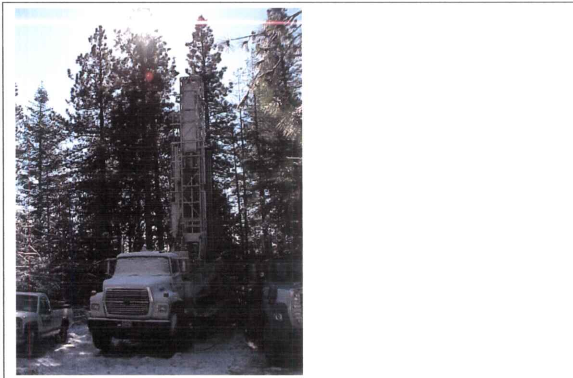
Photo 2: Fogle Pump drilling rig.
