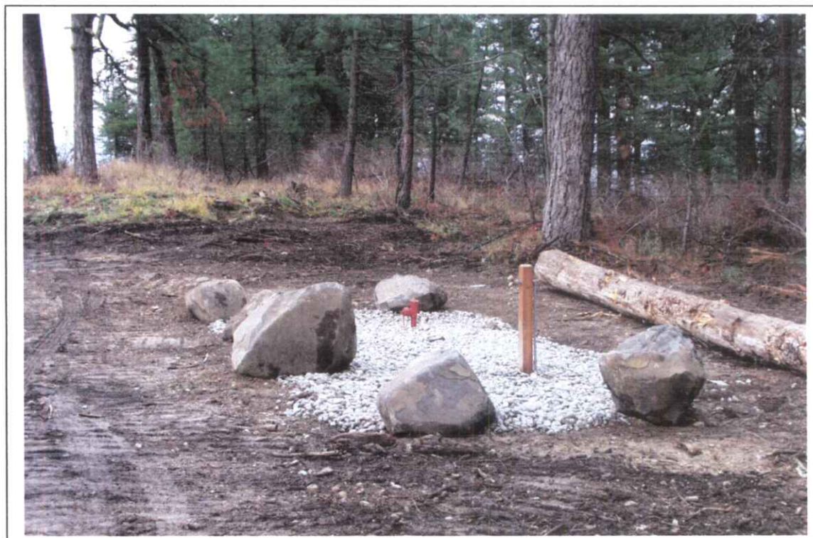
Photo 4: 11-17-04: Spigot and hydrant. Project Completed.
