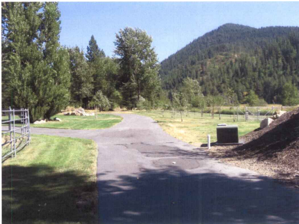
94-7394 East Point of Use are and electrical box
