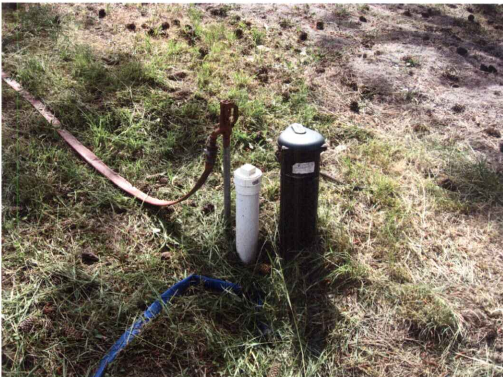
95-9266 Well 2 And Hose Connection to Reel.jpg
