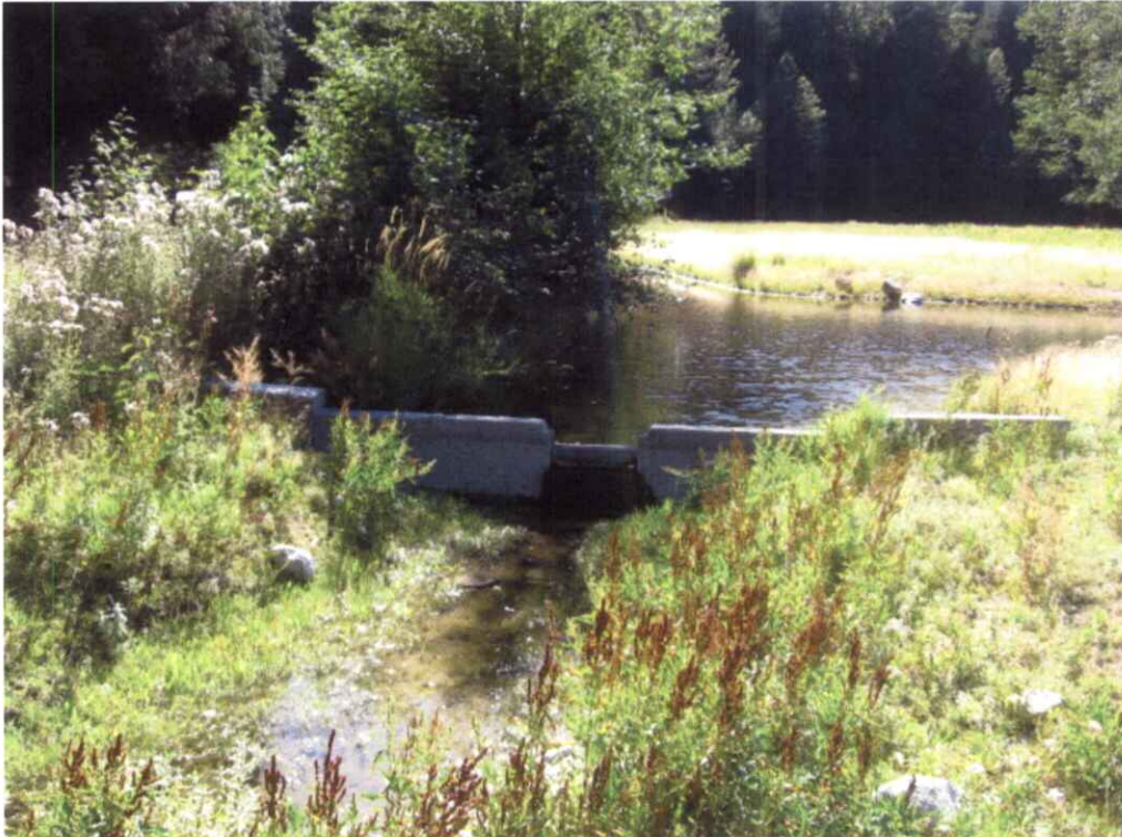
95-9060 Cinder Block Dam With Island Behind
