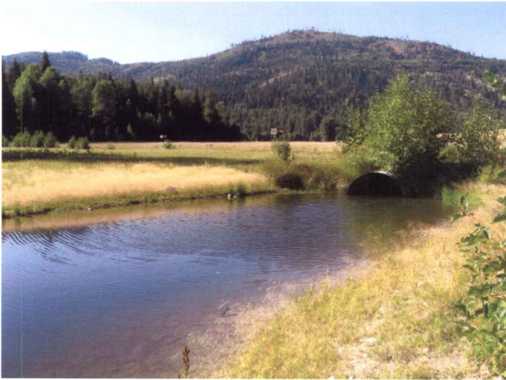
95-9060 Culvert Bridge to Island and Wildlife Nest Platform
