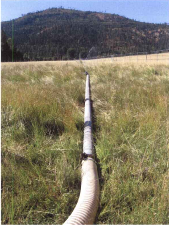
95-9060 Water Line and sprinklers from Pump to POU
