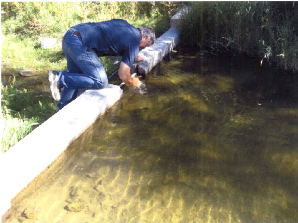
95-9060 Wood Check Boards
