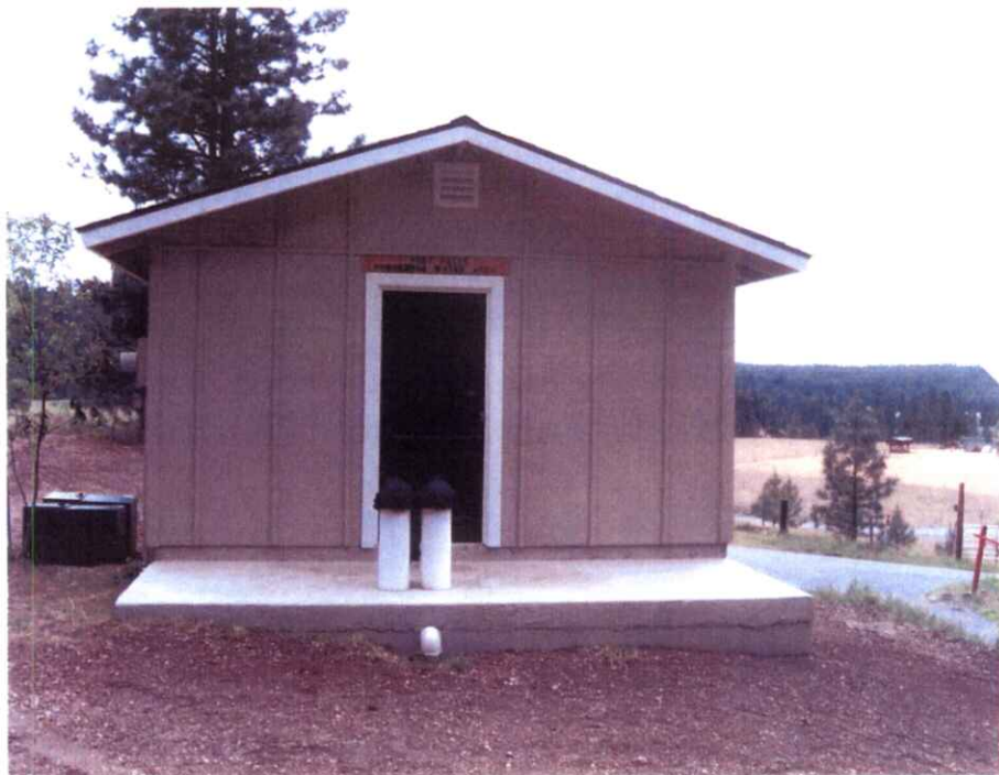
95-9251 Pump House & Partially Buried Reservoir
