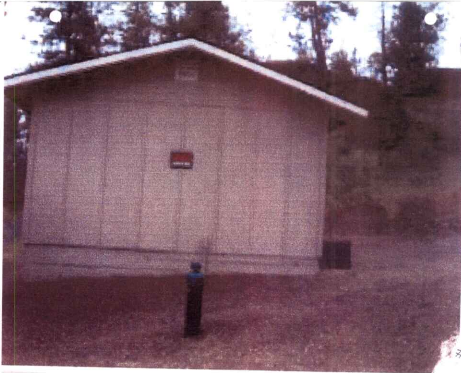
95-9251 Well 2 Behind Pump House
