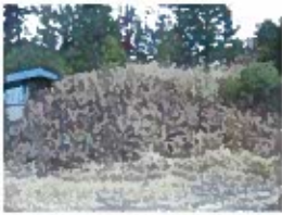
95-8834 earth cover reservoir.JPG
