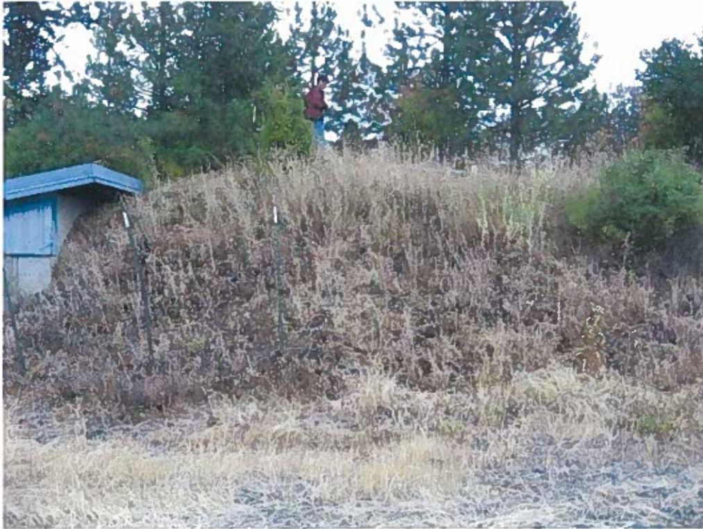
95-8834 Earth Cover reservoirs next to Pump house
