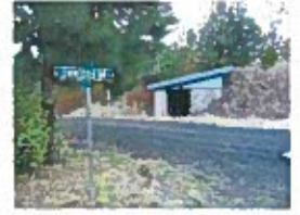
95-8834 Pumphouse & Earth Covered Res.JPG
