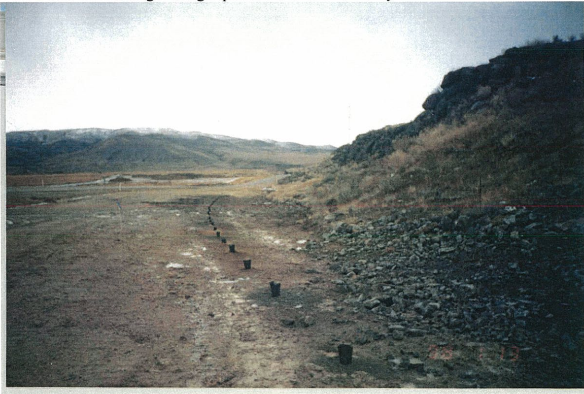
Drill Holes for Blasting During Pipeline Installation January 1998
