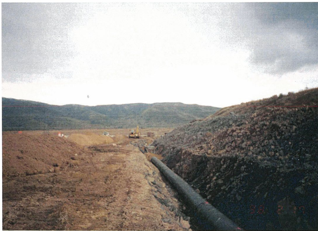
Pipeline Installed in Trench February 1998
