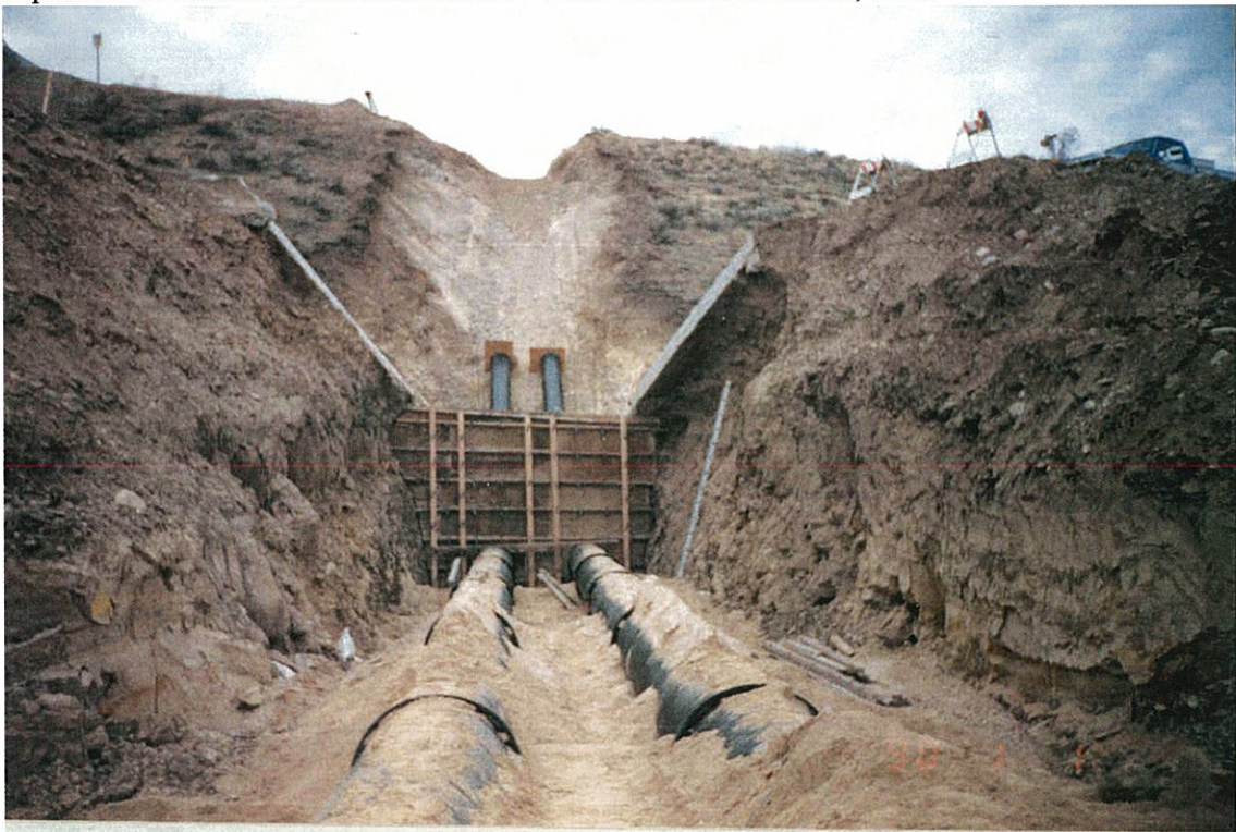
Pipeline Installation Underneath New York Canal December, 1996
