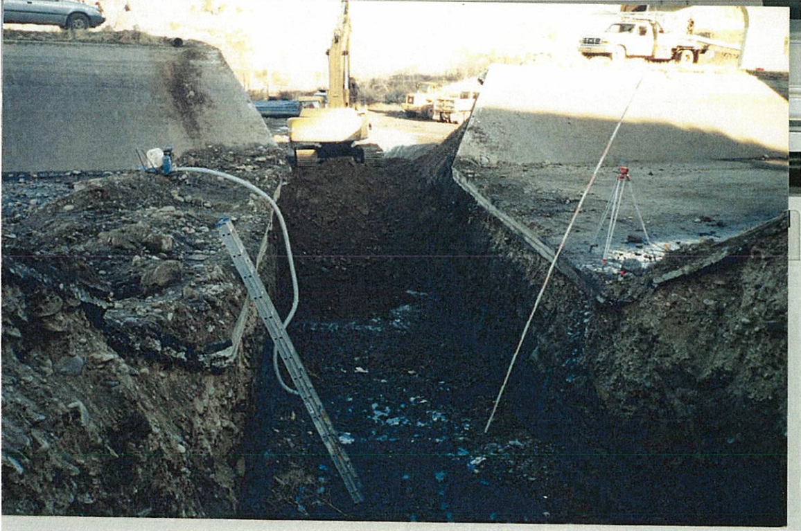
Pipeline Trench Through New York Canal December 1996
