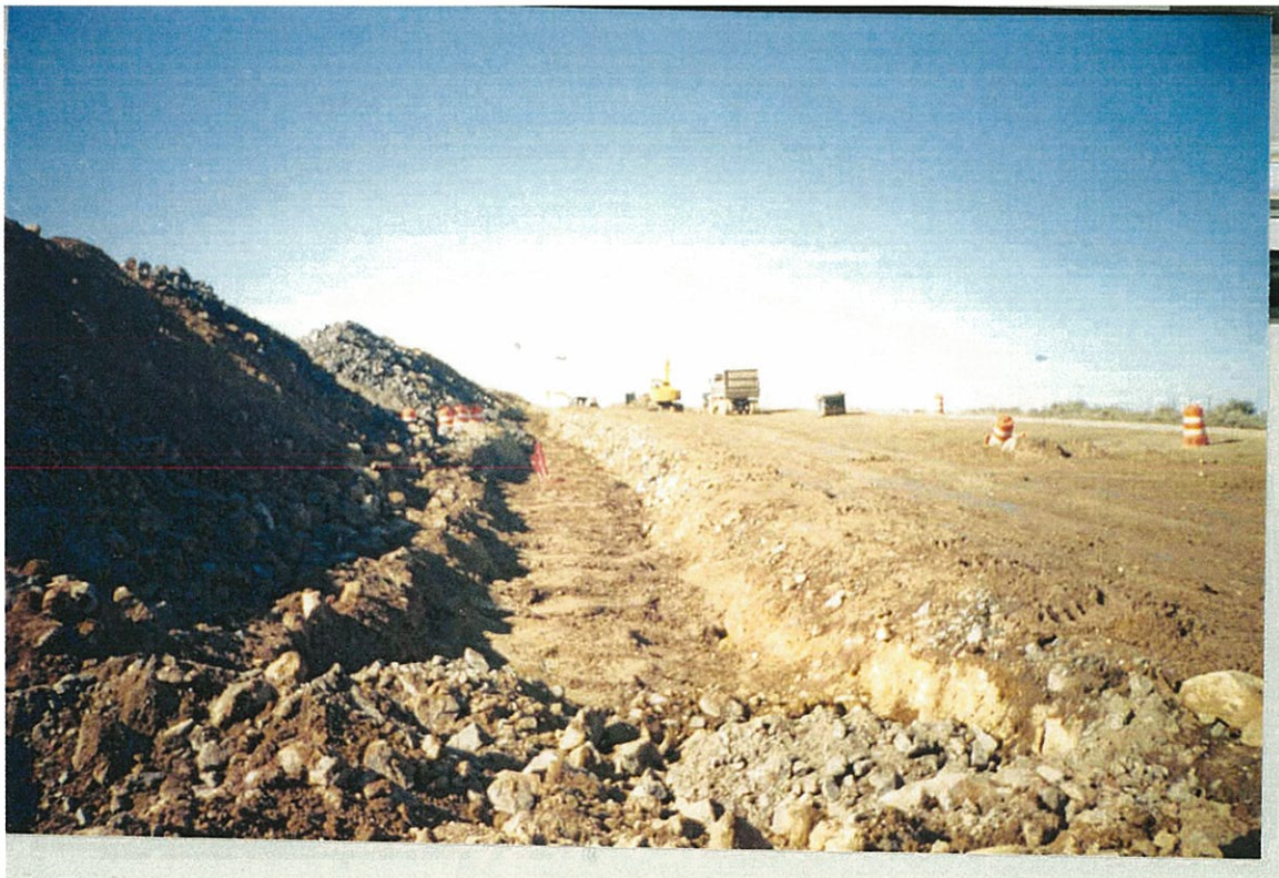
Pipeline Prepared for Backfill March 1998
