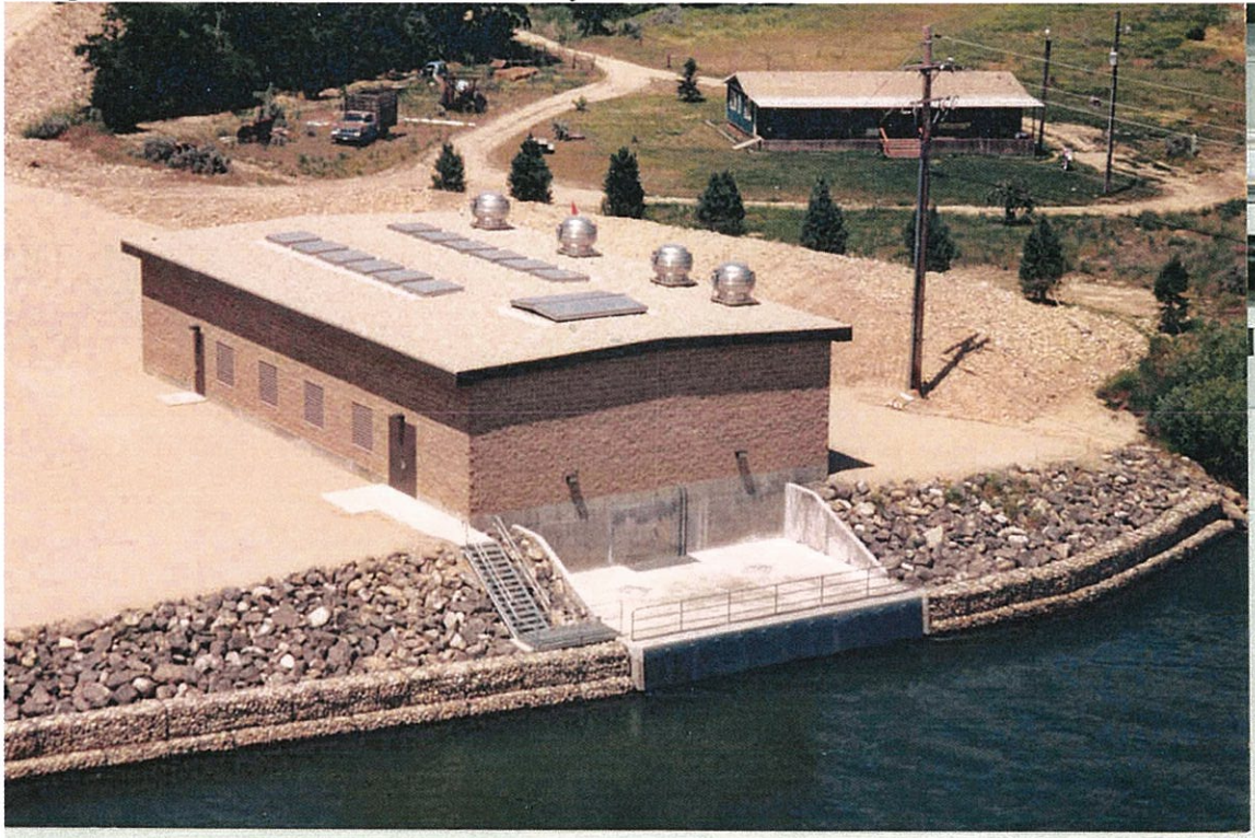
Pump House and Point of Diversion May 1998
