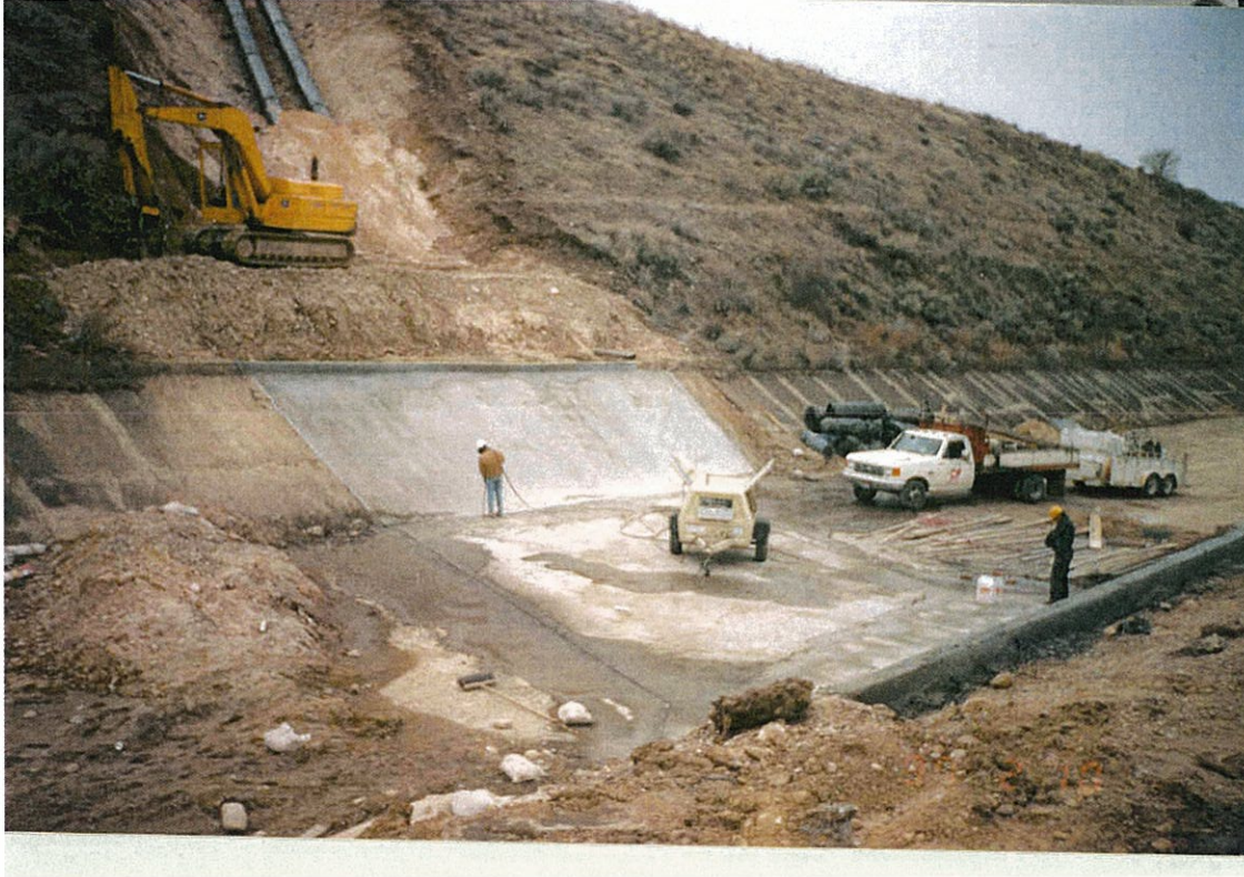
New York Canal Replacement After Pipeline Installation February 1996
