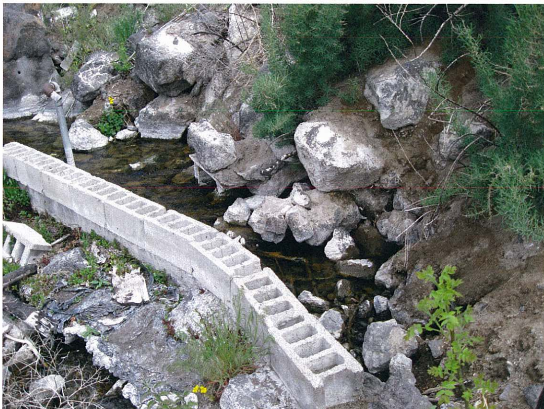
FIGURE 2: Ditch collecting spring water
