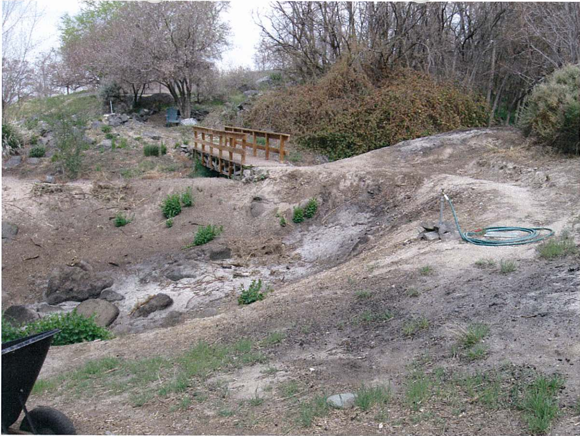
FIGURE 6: Riser pipe with portable hose and upper section of garden and landscaping
