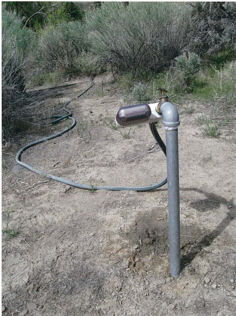
FIGURE 5: Riser pipe with automatic timer control and drip line
