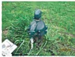
POINT OF DIVERSION
