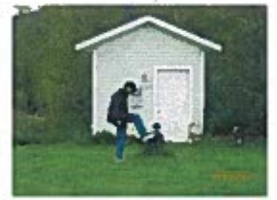
WELL AND WELL HOUSE
