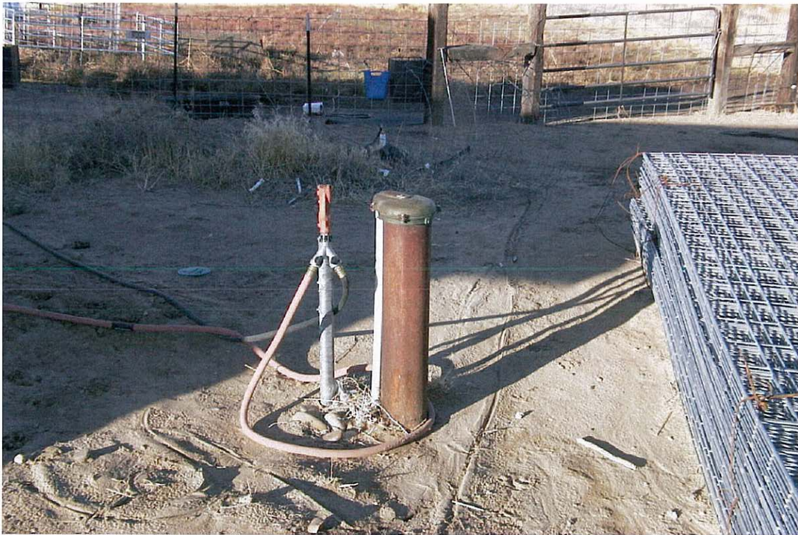
Diversion works—Submersed pump and well location.
