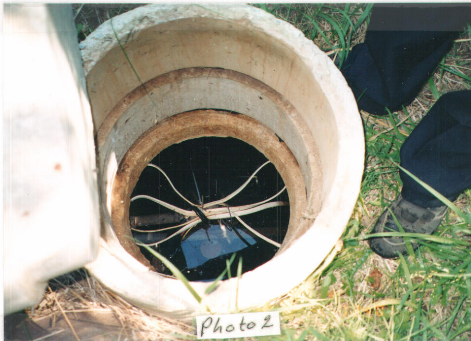
Photo 2. Showing Interior of Storage Tank.
