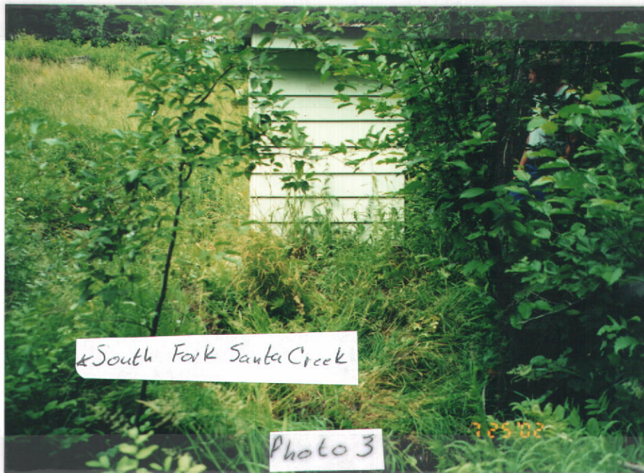
Photo 3. Showing Back Side of Pump House.
