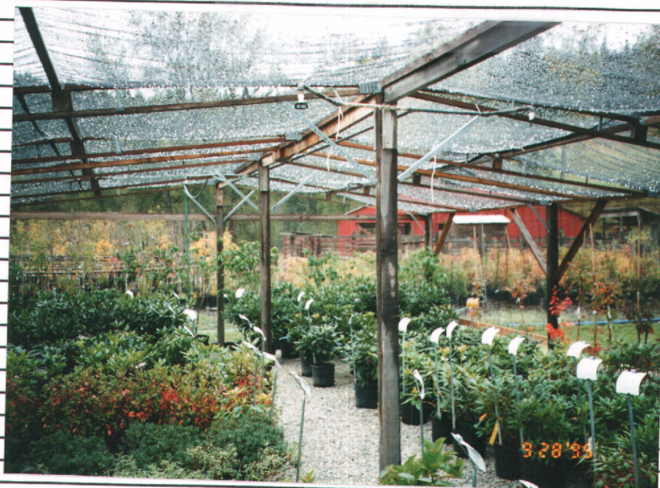
* SHADE HOUSE WITH OVERHEAD "MIST TYPE" SPRINKLERS.
