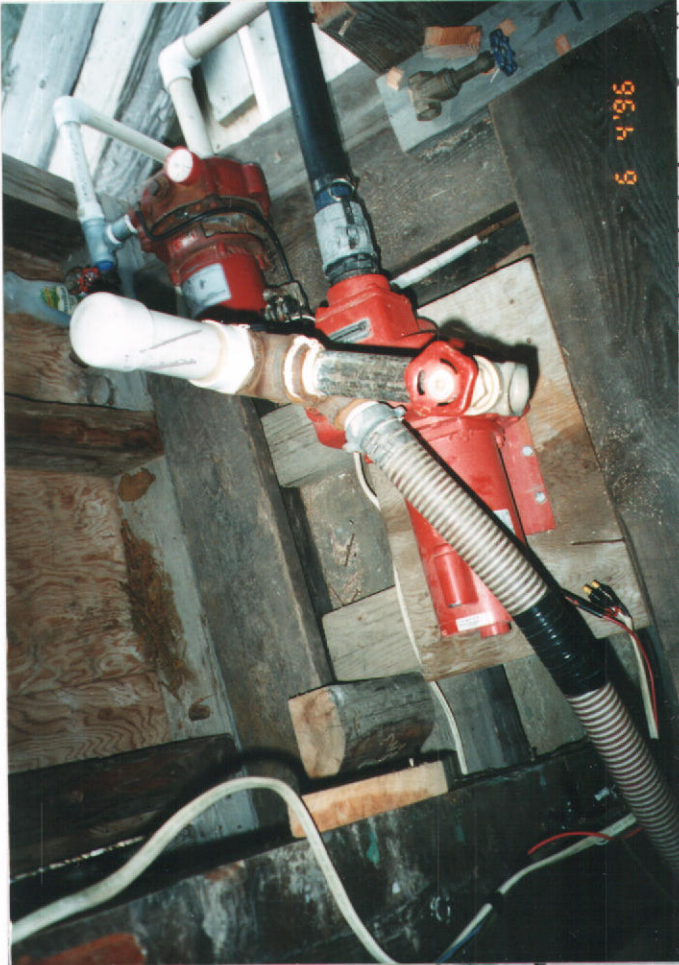
FRANKLIN 2 HP PUMP PUMP SITE
