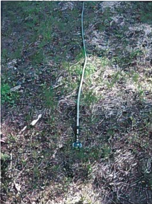
95-9166 Irrigation hose to grassy lot West of house
