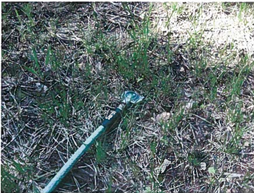
95-9166 Sprinkler head close-up grassy lot West of house
