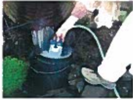
Submersible Pump at POD.JPG
