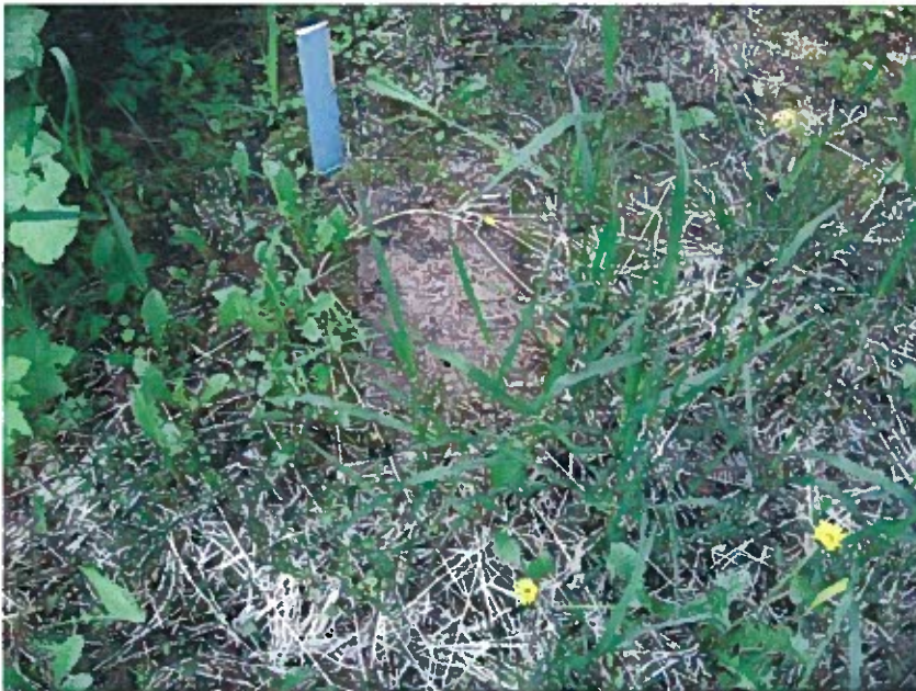
95-9166 Lid for Kidd Island Bay water line
