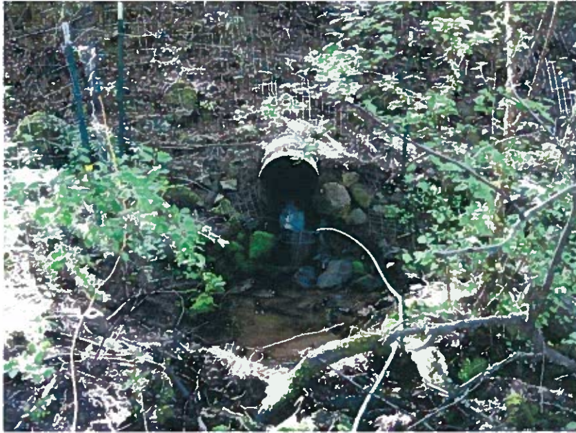
95-9166 Point Of Diversion (POD) on unnamed stream
