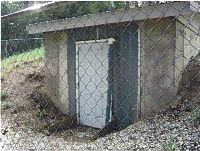
95-8684 Well 3 at reservoir
