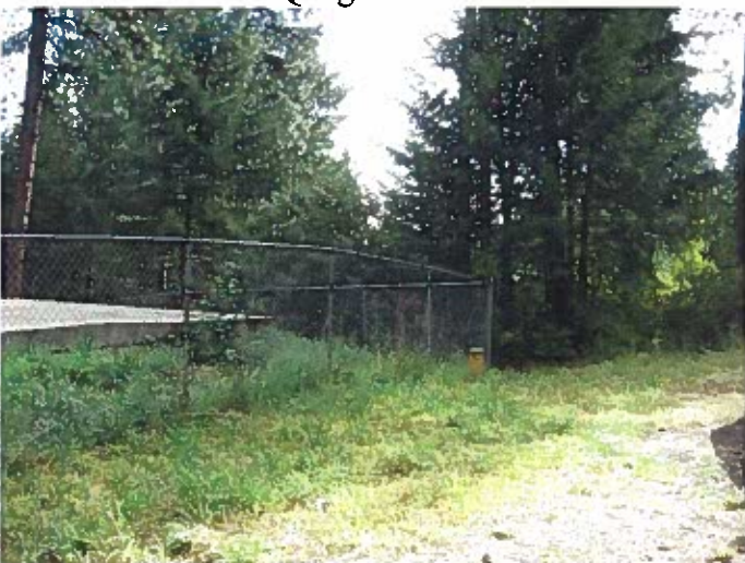
95-8684 Well 3 location at reservoir
