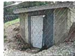
95-8684 Well 3 at reservoir.JPG
