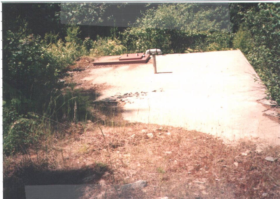
CONCRETE STORAGE TANK & LOOKING N. WESTERLY
