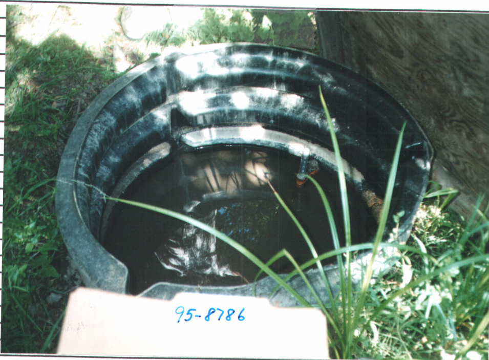
Point of diversion
