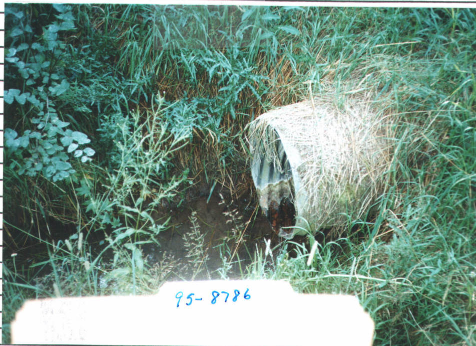
Point of diversion
