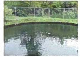
92-7171 Sand Filter Center Overflow Pipe.jpg
