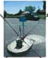
92-7171 Drinking water at RV site.JPG
