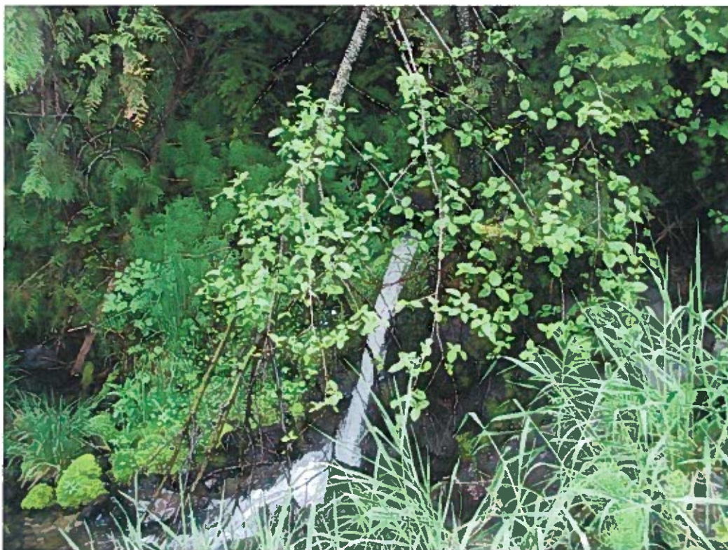
92-7171 Overflow to Finn CR before flowmeter test.jpg
