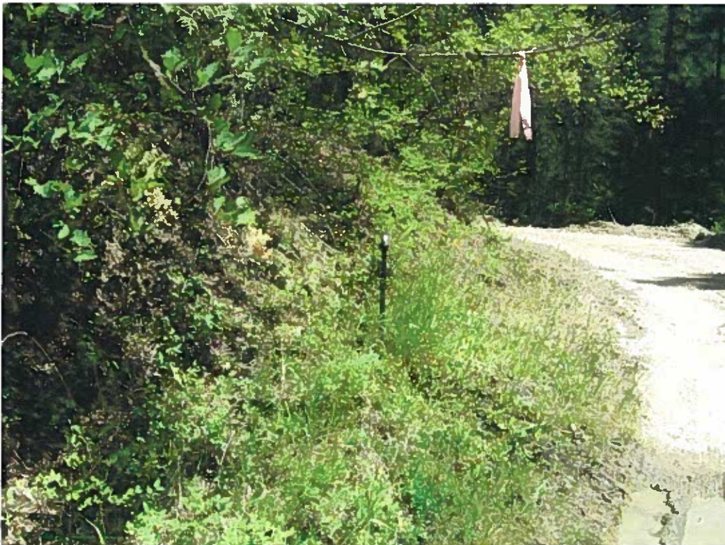
92-7171 Pipeline Breather on Dale DR.jpg
