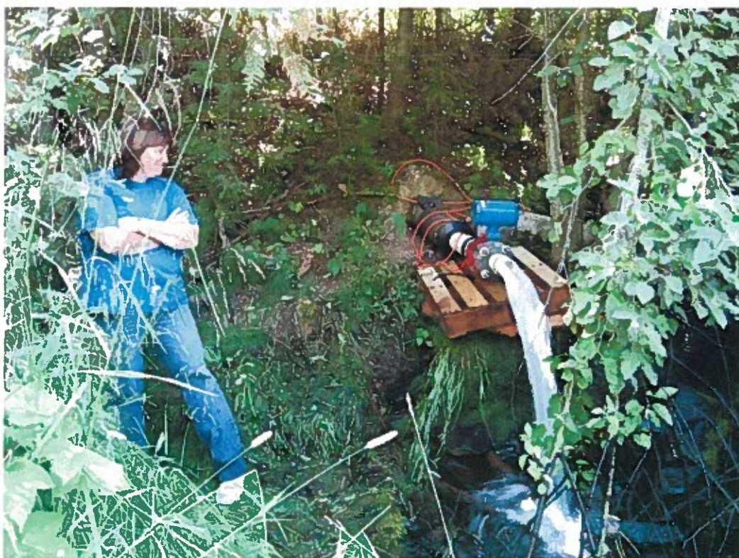
92-7171 Overflow to Finn CR Flowmeter Test.jpg
