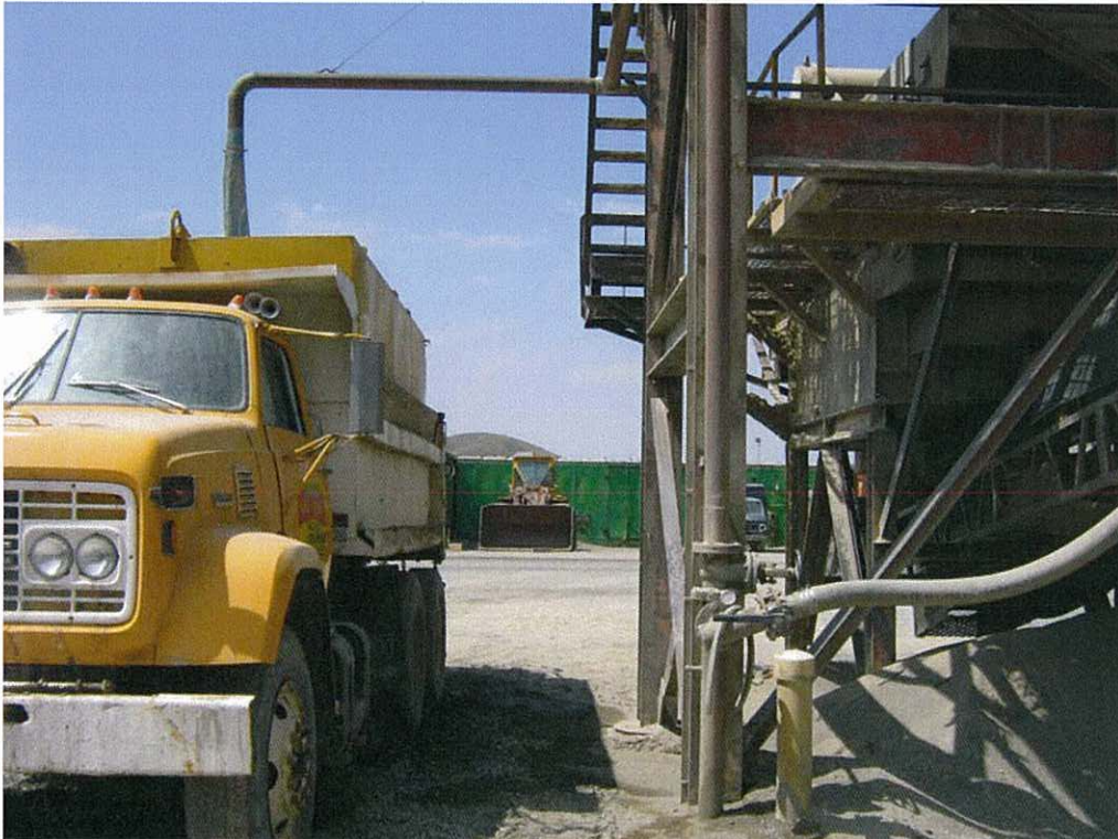
Truck Filling Station
