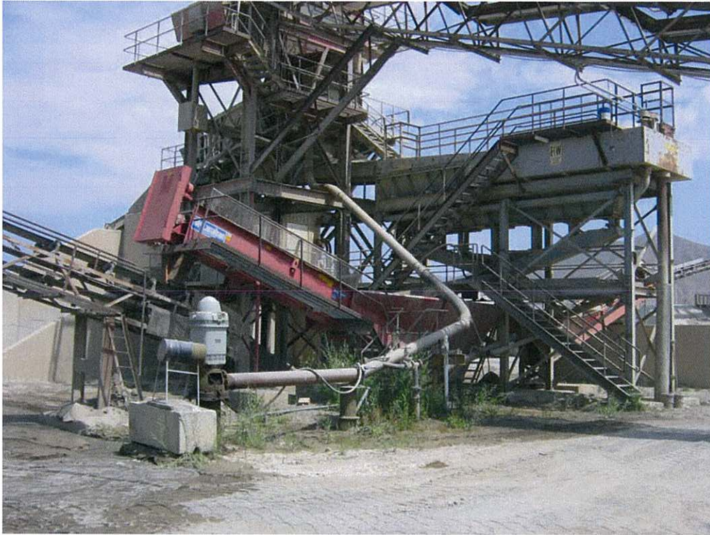
Crusher Well, 10" Pipeline, Sand Separator & Classifier North
