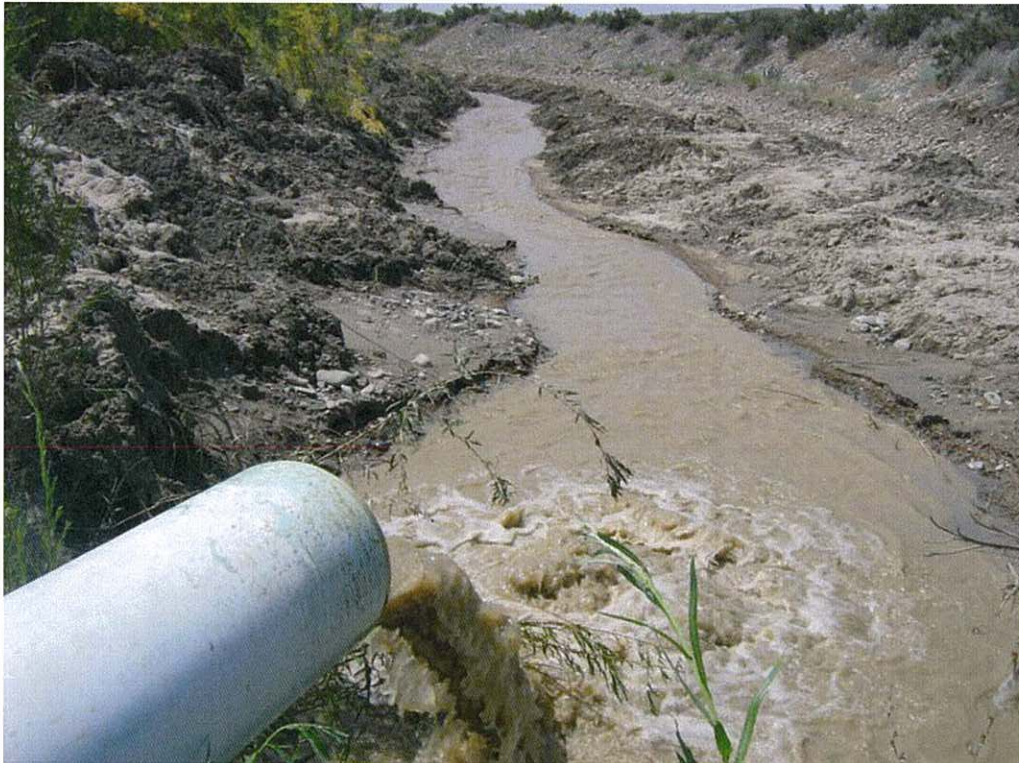
Wastewater Pipe Discharge
