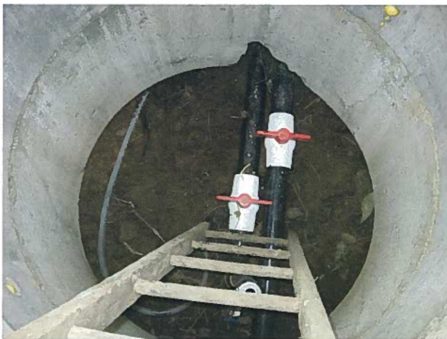
95-9120 Vault Interior AUG 2007
