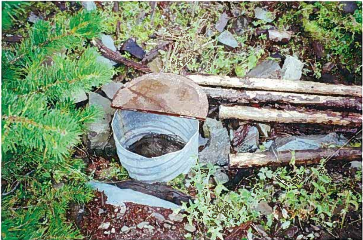
headbox just above road in ditch
