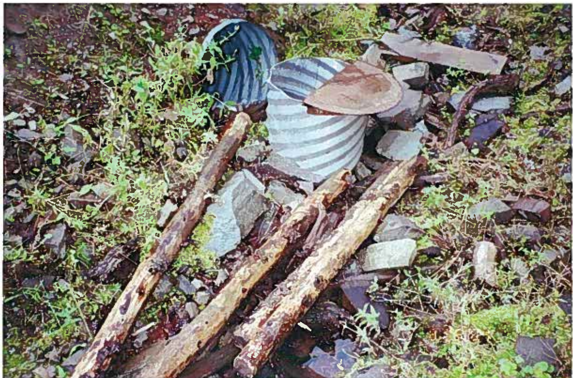
headbox just above road in ditch
