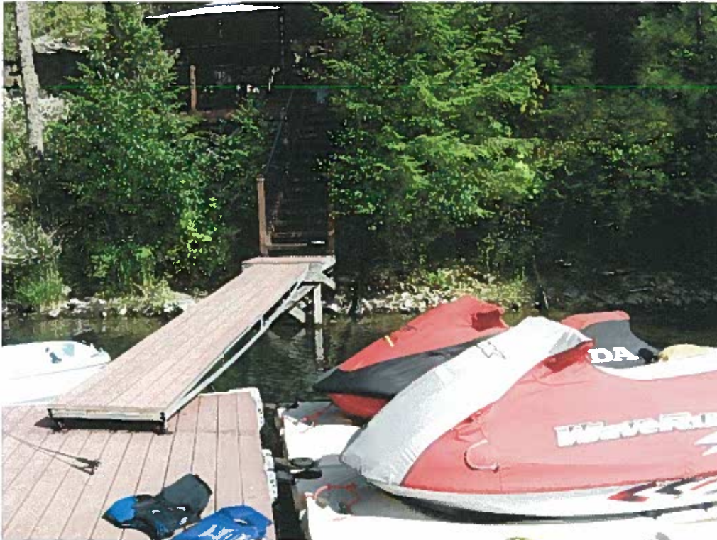
95-9352 Two Inch Water line climbing out of Hayden Lake
