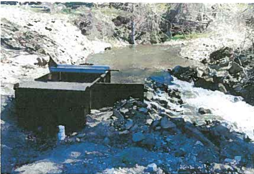
Kenney Creek Diversion #3 (Kenney Crk PL)
