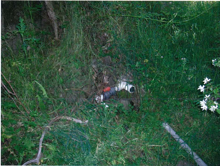
Perforated drain pipe has been installed 10' "back" into the hill and spring. End of drain line is capped, line coming off of the "tee" fitting is valved and connects to a 2" poly line that drains to a 600 gallon tank. Gray pipe in lower right hand corner is actually a hand made "roto-roooter" auguring tool used to maintain the drain pipe in the spring.
