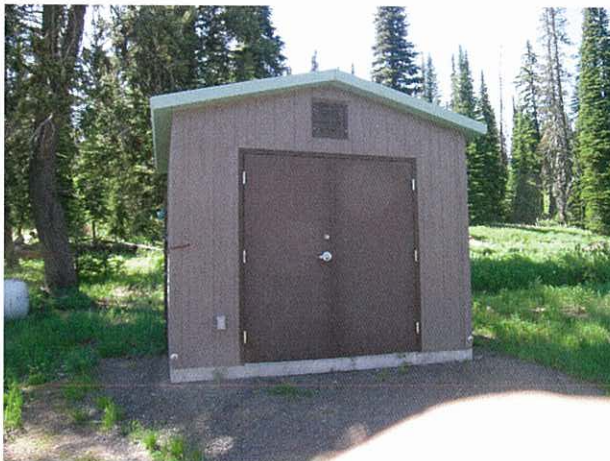
Hard Creek GS Utility Shed
