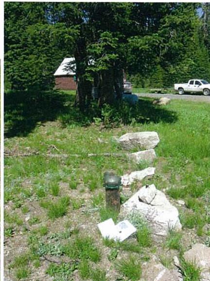
Well w/ GS in background.
