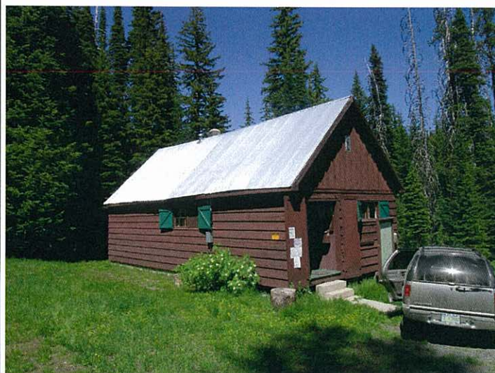
POU, Hard Creek Guard Station
