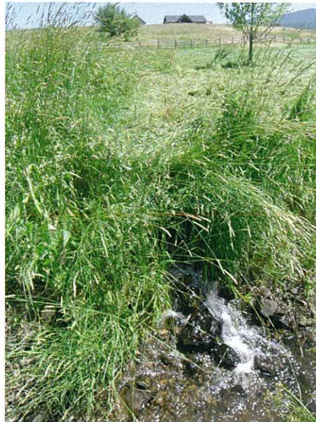
Open Channel Pond Outlet Discharge Point.
