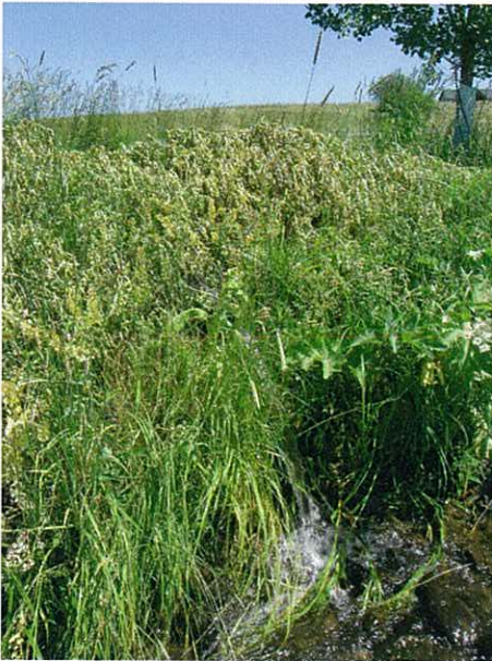
Piped Pond Outlet Discharge Point.
