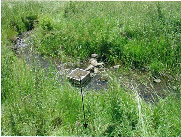
Screened Inlet Device in Johns Creek.
