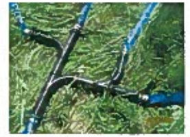
SPLITTER FOR FLOOD IRRIGATION.JPG
