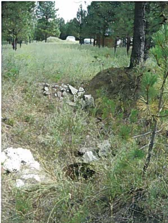
BWS- Non-System Reservoir BLDG & Valve
