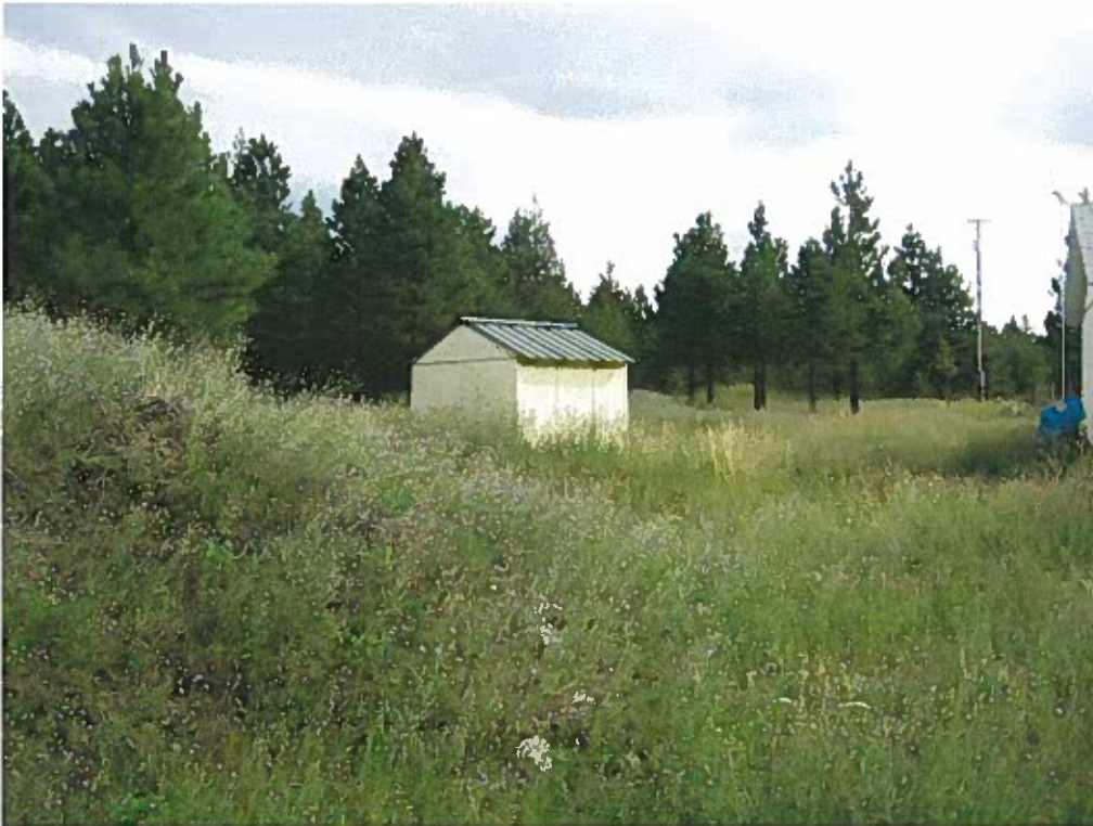
BWS – Non-System Reservoir BLDG & POU
