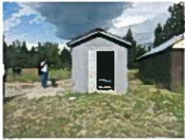
BWS Well Location.JPG
