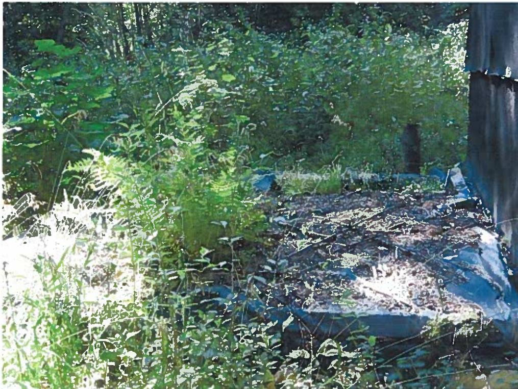
95-8999 Pumphouse with reservoir
