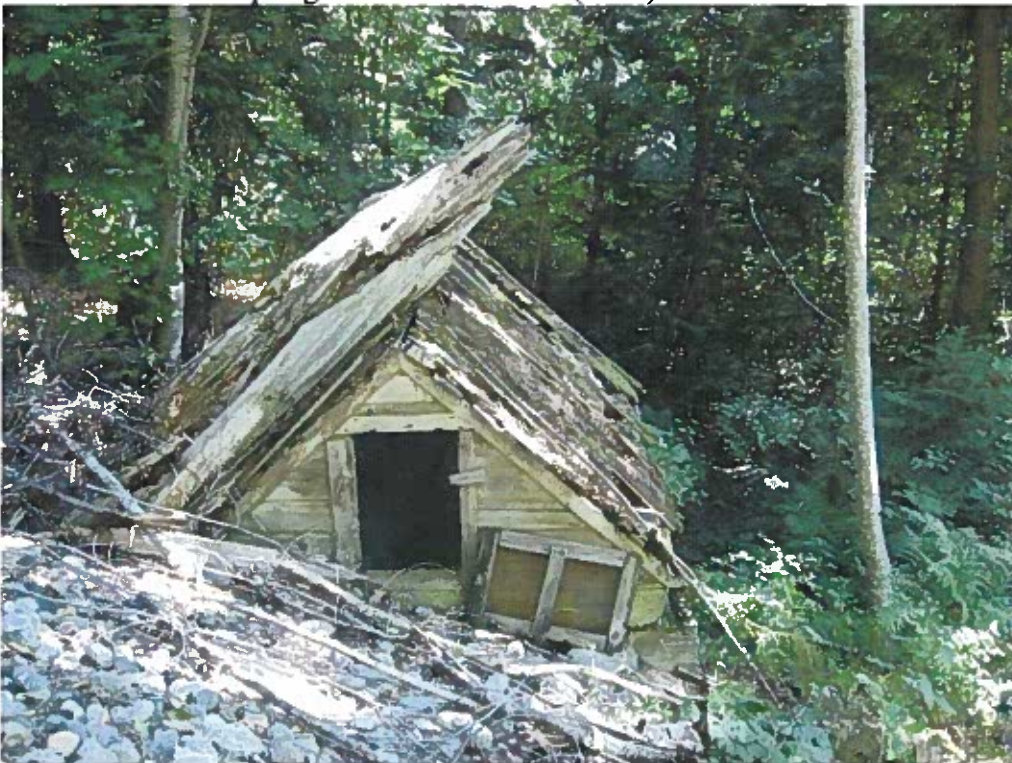
Old Pumphouse not 95-8999
