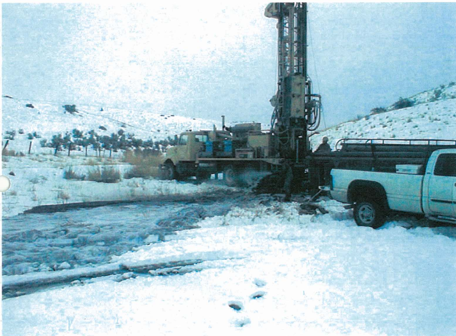
DRILLING OF SPRING VALLEY EXPLORATION WELL SVR 5 JANUARY 20, 2004 ADAMSON PUMP AND DRILLING air-rotary method; note gray drilling foam in the foreground
