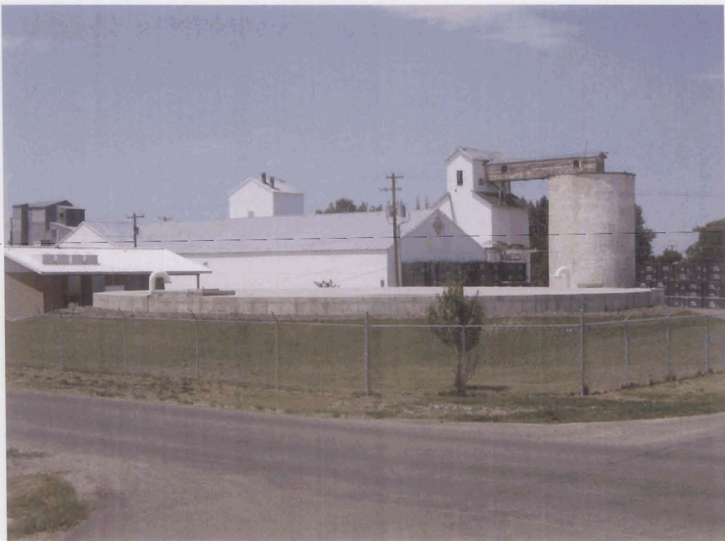
New Pump House
