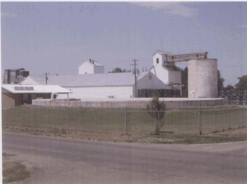
New Pump House
