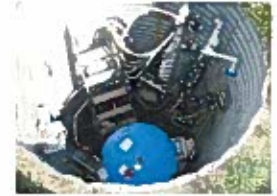
95-8998 Steel Vault Interior.JPG
