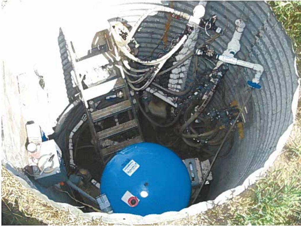
95-9889 Well Vault (Steel) Interior
