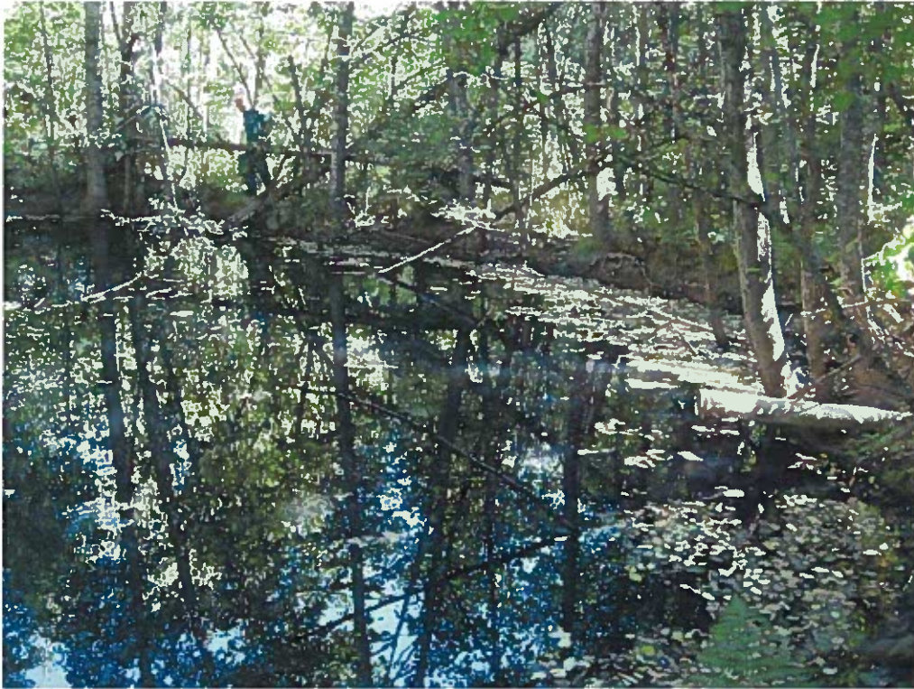
95-8998 Pond Pipes Not Connected
