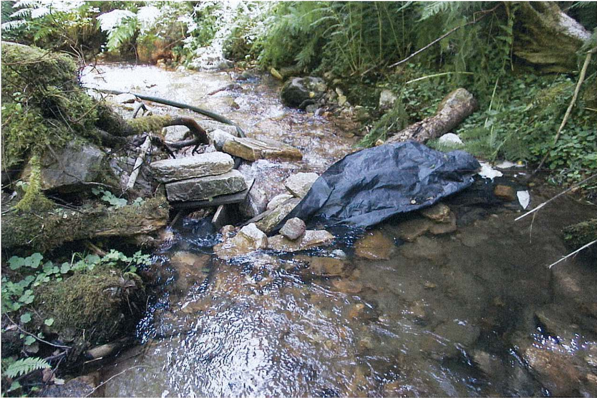
FIGURE 1: Diversion dike and box, view facing downstream.
