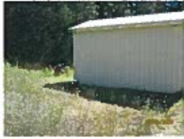
PUMP HOUSE 2.JPG
