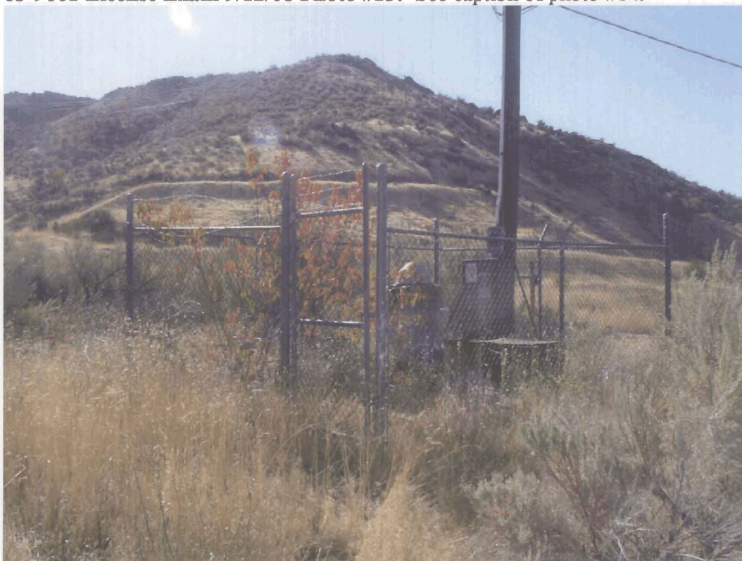
63-9661 License Exam 9/12/08 Photo #16: Old Penitentiary Well #1 previously on permit Well currently not in use.
