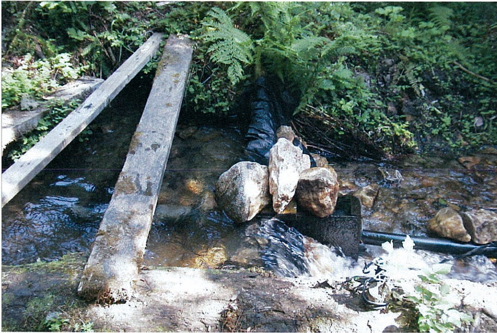
FIGURE 1: Diversion dike, box, intake, and pipeline. Downstream is to the right.
