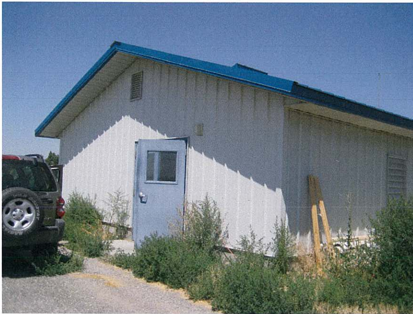
Pump House for City of Bliss
