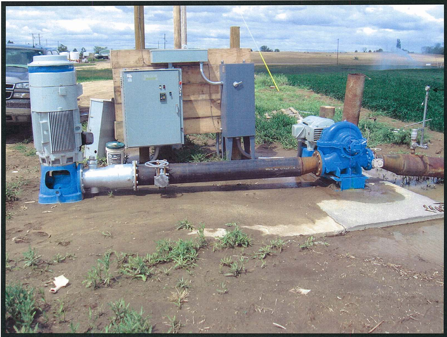
16" East Well, 150 HP Pump, 125 HP Booster
