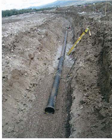
Installation of water line on going
