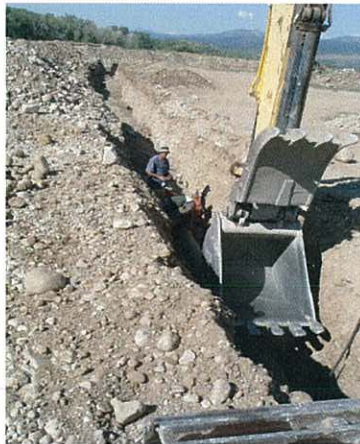
Installation of valve network near MH#7 for water main
