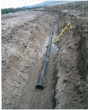
Installation of water line on going
