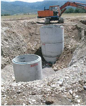
Compaction of lift station
