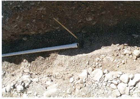
Pressure sewer with bedding
