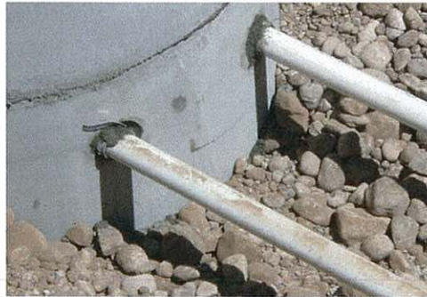
Lift station lines, Note grout
