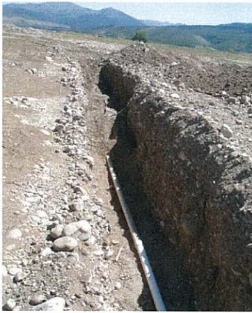
Pressure sewer with 24 inches of 1" minus
