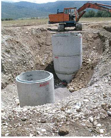
Compaction of lift station
