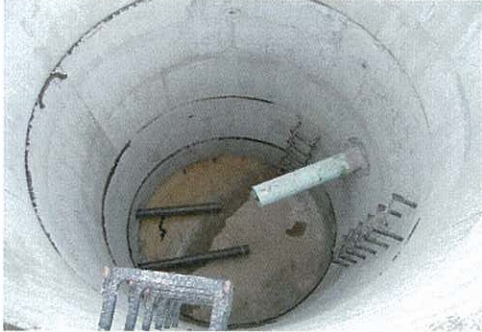
Picture looking down into sump
