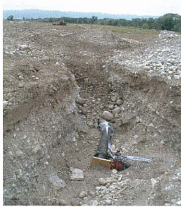
Water line showing trench fill Compaction by wheel rolling
