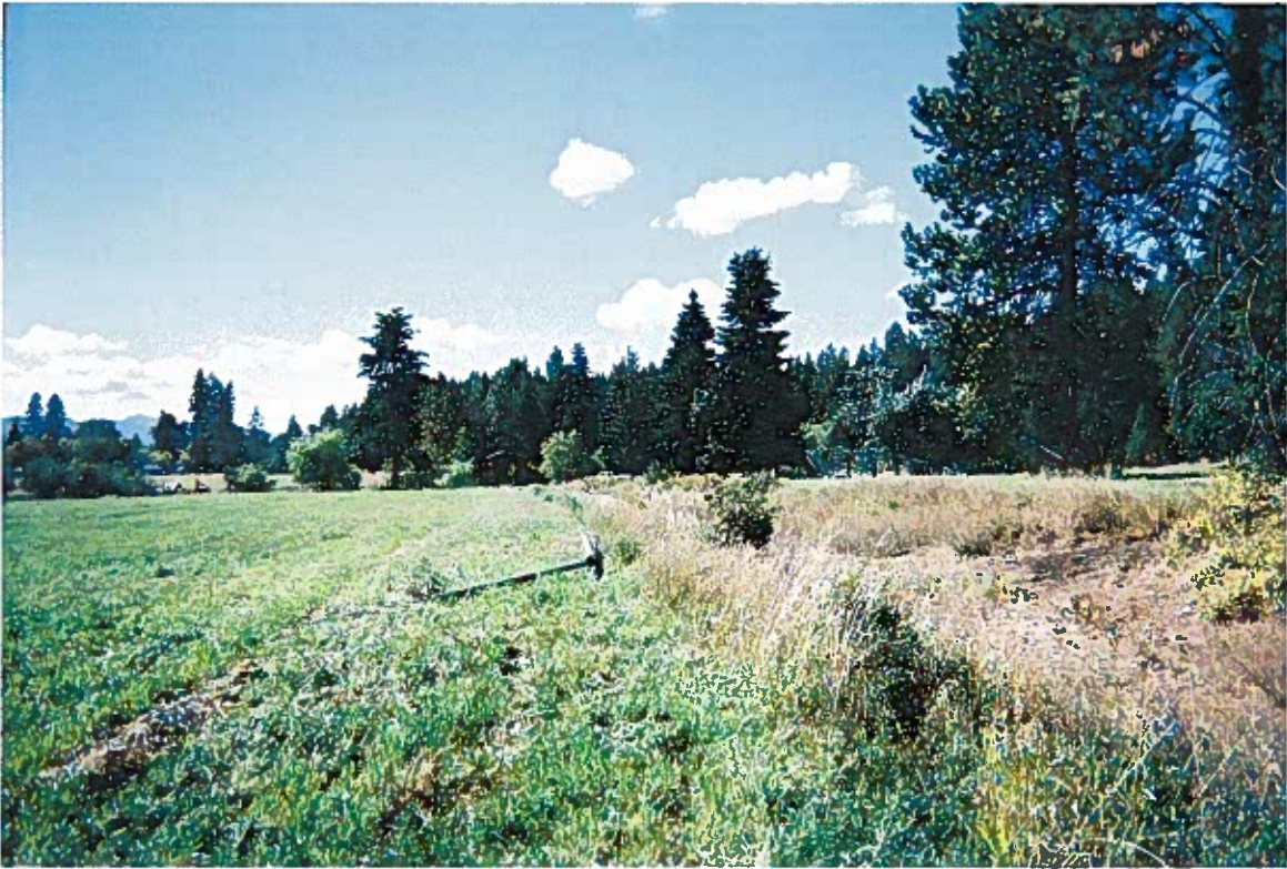
95-8858 North POU Handline R & Pipeline L
