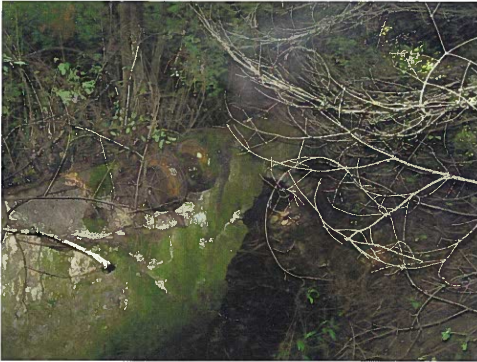
95-8457 Dam 1 Hole AUG 08
