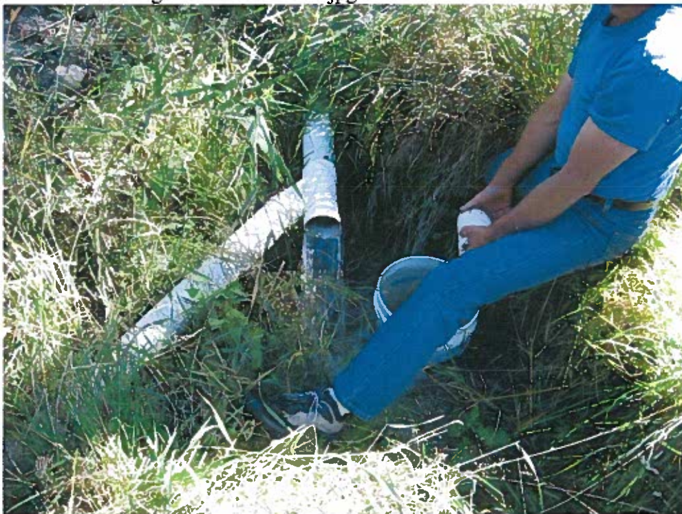
97-7276 Flow at 1 st Elbow From POD.jpg
