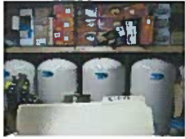
inside pump house.JPG
