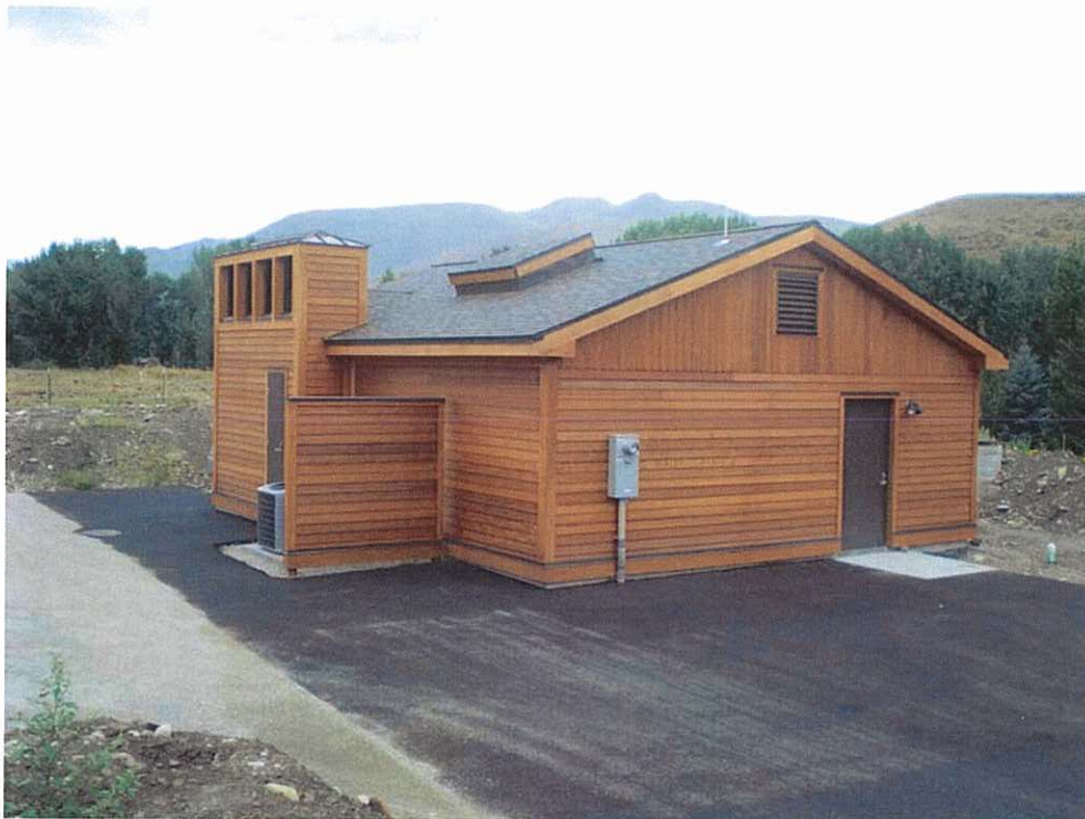
Sun Valley Water and Sewer District "Well 12"
