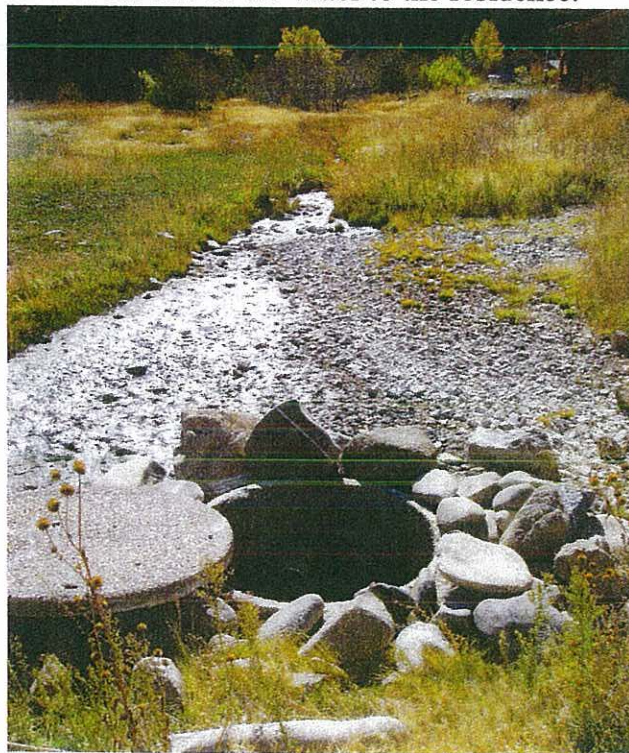
Photo 5. The Pace standpipe is visible in the foreground with surrounding alluvium visible. The muddy area surrounding the standpipe is covered with water when the standpipe operates at “high” water level condition
