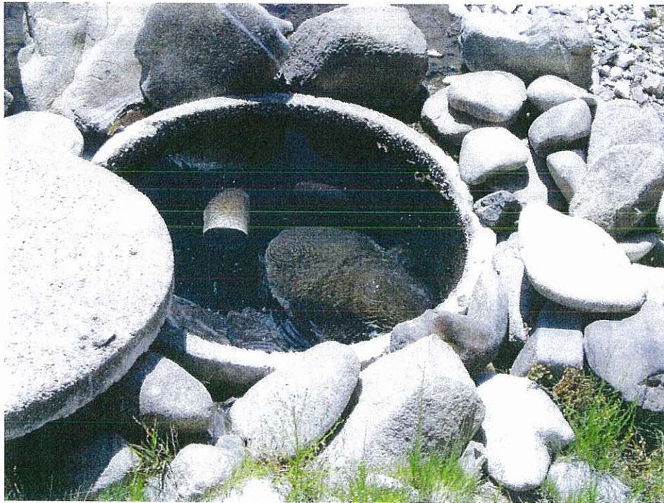
Photo 2. Pace collection system (standpipe) at “high” water level operational condition.
