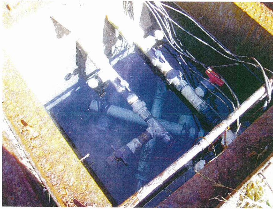
Photo 3. The Robbins sump collects water captured in perforated pipes, and submersible pumps located near the bottom deliver the water to the residence.
