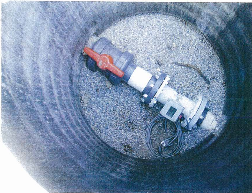
Photo 8. Robbins system magnetic flow meter. IDWR staff took hourly readings from this meter to track Robbins pumping rates.
